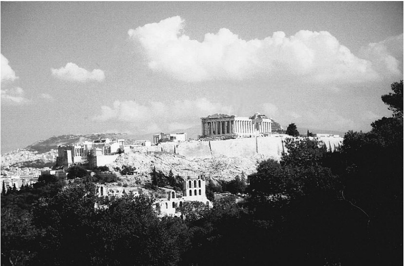
Figure 11. Athens: acropolis; Propylaea to left, Erechtheum in background, Parthenon to right (all second half of fifth century), Odeum of Herodes Atticus in foreground (second century AD).
