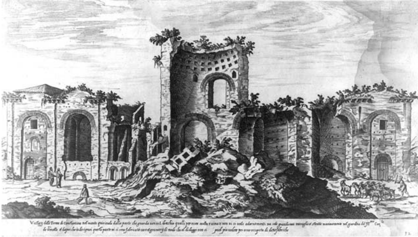
FIGURE 33. Baths of Constantine on the Quirinal, Rome. Engraving by E. Du Pérac 1575. Fototeca Unione no. FU 4769. Copyright Fototeca Unione/American Academy in Rome.
