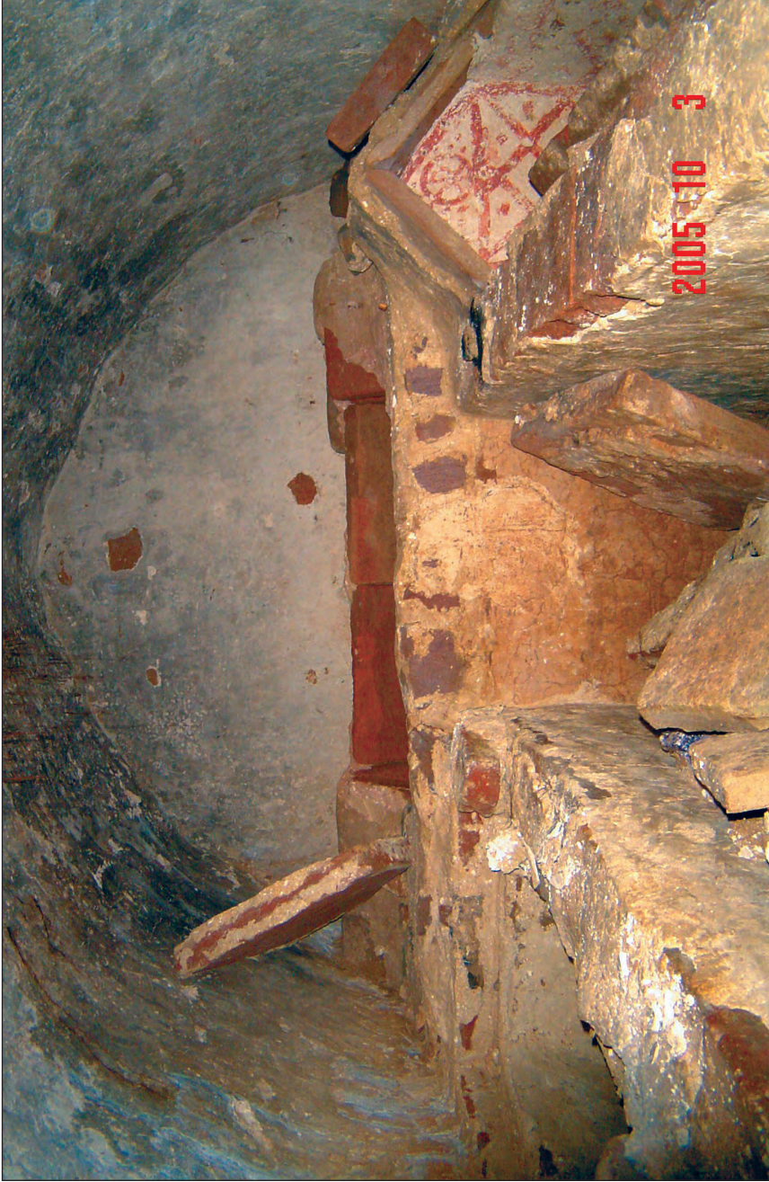
Figure 5. Burial chamber XX was plastered, but unpainted. The grave is against the back wall, two secondary graves to the right and left made with different building methods. © Zs. Visy
